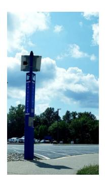
The college has 6 Emergency Blue Light Towers installed around the main campus. Each tower is blue with a white "EMERGENCY" label and a blue strobe light on top. The blue light activates when the "HELP" button is pushed and released. This triggers a call to Campus Police where you can report your emergency. Officers will immediately respond to assist with the emergency.
