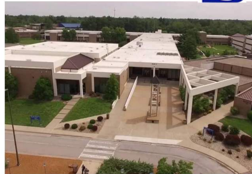
Existing main entry
