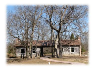
The Harrison Storefront is divided into two pens, one on each side of the concrete-floored breezeway or "dog trot". Entry into each of the two pens is gained by way of the dog trot through a door in the center of each of the inner walls. In pioneer times, this floor plan provided a way of separating the kitchen, with its eternal fire, from the living quarters during summer months. It also provided for a covered passage between the two pens during inclement weather.
