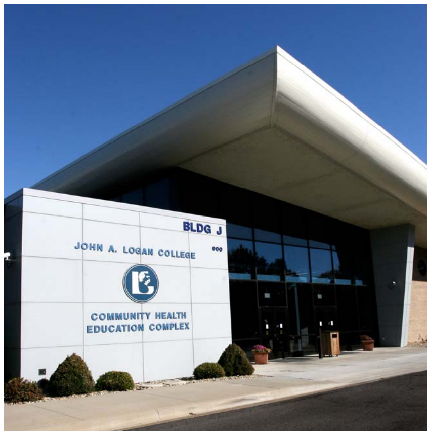
Community Health Education Complex (CHEC) Building
